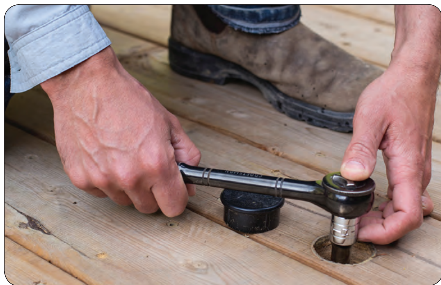
Level any deck from the top with the simple turn of a ratchet.
