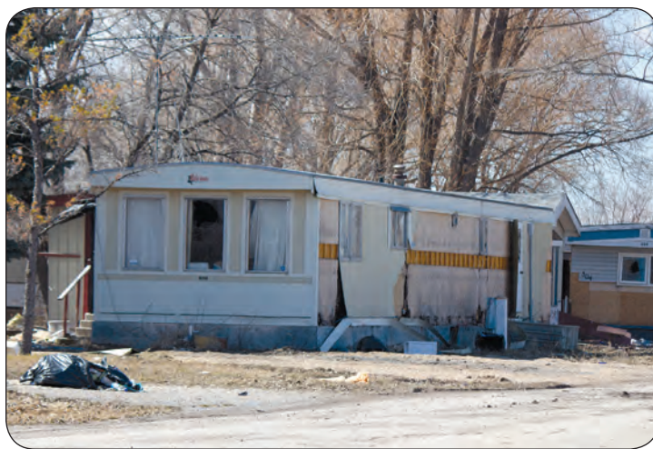
An abandoned mobile home and a large pile of debris are pictured at the former site of the Selkirk Trailer Park on April 17. According to a sign posted outside the park, the developers say the park will be demolished no later than May 30.
