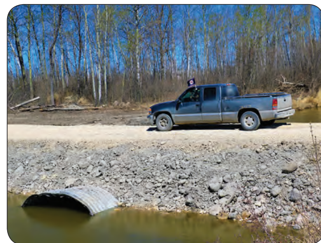
Minor flooding from ice jams this spring entailed the removal and replacement of this crossing over the Fisher River near the Pine Cone Dairy Bar.
