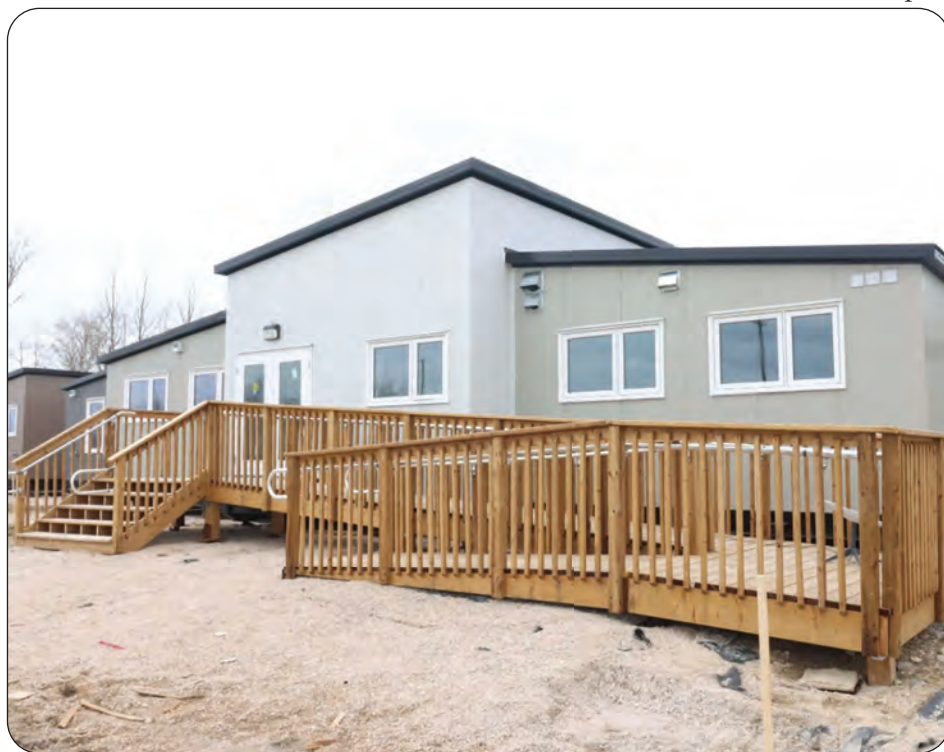
Bison Modular Homes recently completed a women's shelter in Lake Manitoba First Nation.
