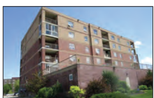
1404-6940 Henderson Hwy, Lockport $279,900
